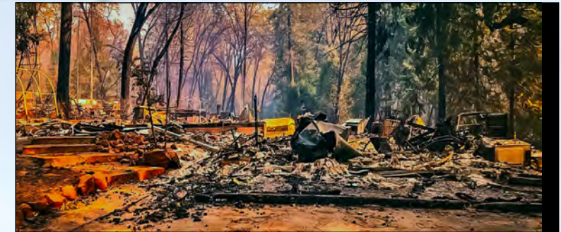
The remains of the Stroud home in Magalia after the fire struck on November 8. The Strouds were fortunate to escape with their children and pets, but, unfortunately, little else. They are staying with family in Vacaville. The Strouds are overwhelmed with the caring support of the community.
